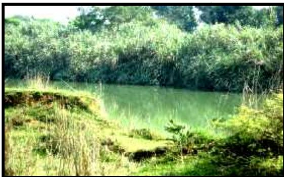
Maintenance of embankment by applying the local technology: Vegetative treatment in 300 fit earthen river embankment has been maintained by plantation. River embankment was covered and protected by Humiculata and Cane grass almost 4 km of area.
